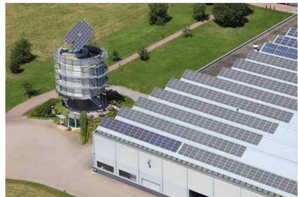
Solar power plant in Offenburg: 20 years ago Hansgrohe installed Germany’s then largest roof-integrated solar power system at its production site in Offenburg
