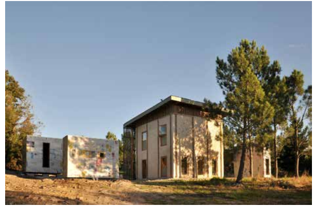
The new sanitation pavilion at the "Village of Hope"
