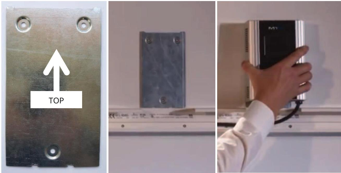
To fix it to the wall bracket, the AC•THOR is suspended in the wall bracket by the two long slots on top and then fixed in place by locking it underneath (slide to the left).
