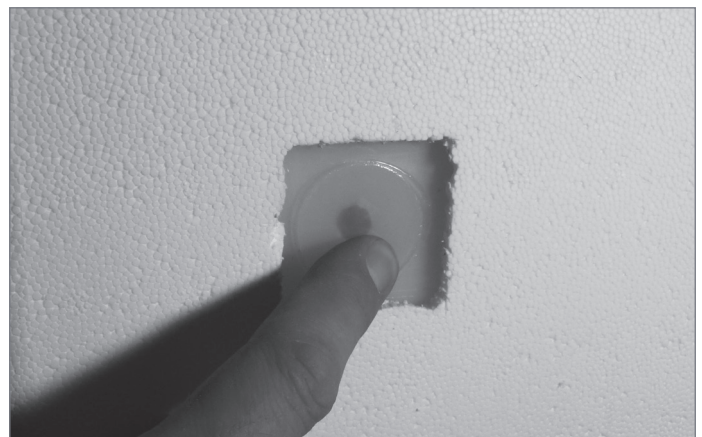
6. Put plastic disc directly on cistern and press short-time
