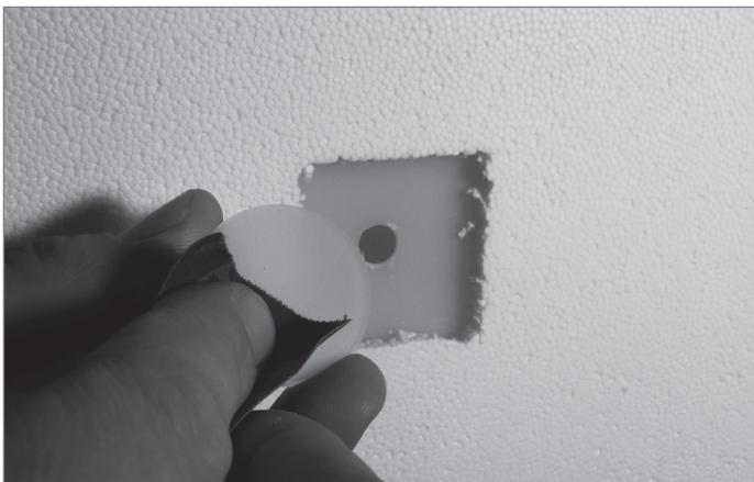
3. Roughen both glue areas with abrasive paper
