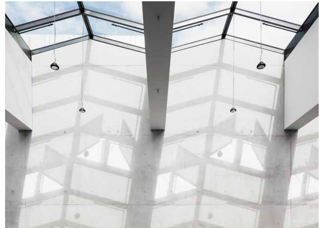
A multifunctional venue for trade fairs, The CityCube in Wilmerdorf gives a sense of air and lightness despite its impressive size of 23,000 square metres.
