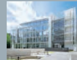
GROHE Firmenzentrale | Headquarters Düsseldorf | Düsseldorf
