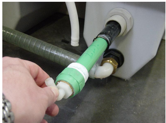
Removing the aerator unit
