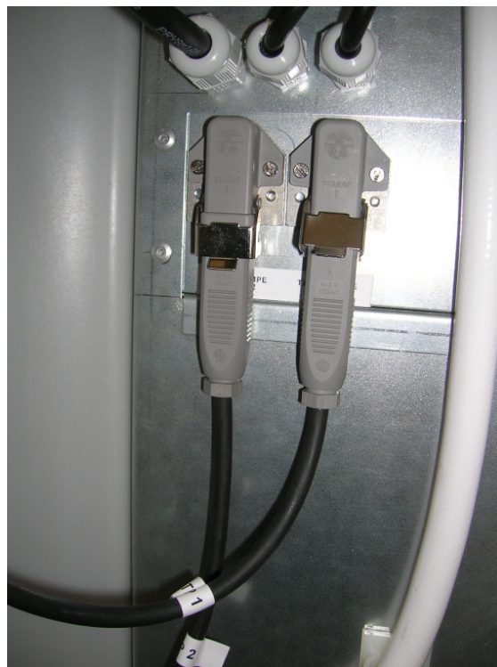
Conector bombas sumergibles
