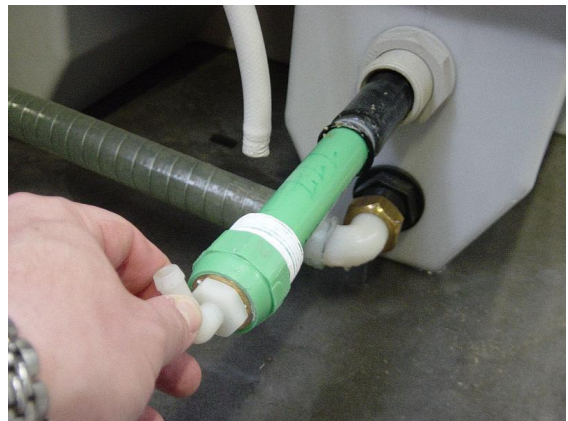
Removing the aerator unit
