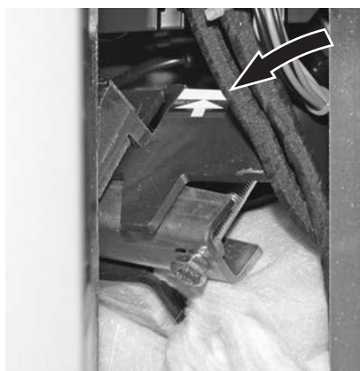
Fig.12 Tighten fastening at top as firmly as possible (as marked)
