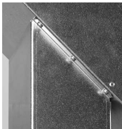
Fig.23 Secure pedestal at the sides with 3 screws each
