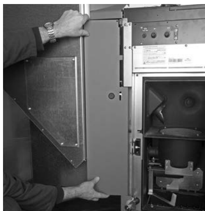
Fig. 34 Insert front cladding
